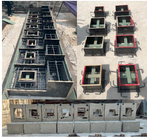
Figure 2: Pre- and post-fabrication of the FDPC deck; and formworks of shear pockets with steel angle confinement.
